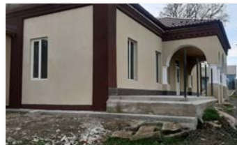
Exterior close to its finish
