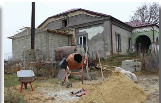
A Work In Progress
