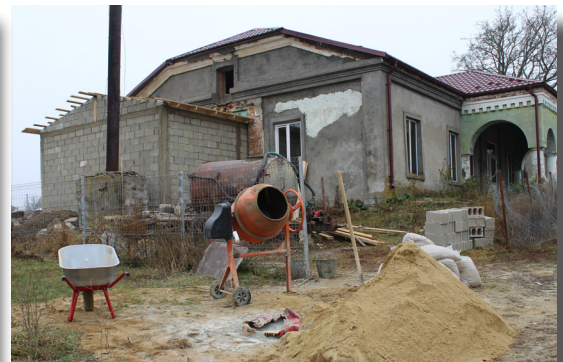
A Work In Progress
