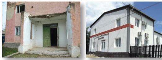
Town of Colibasi Recreational Center...BEFORE & AFTER
