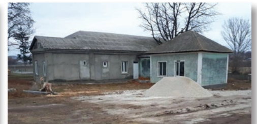
Backyard grading begun
